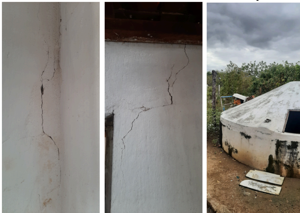
Figures 3, 4, and 5: Images of cracks recorded on the house walls and cistern of a resident of the Quilombola Pitombeira Community.
