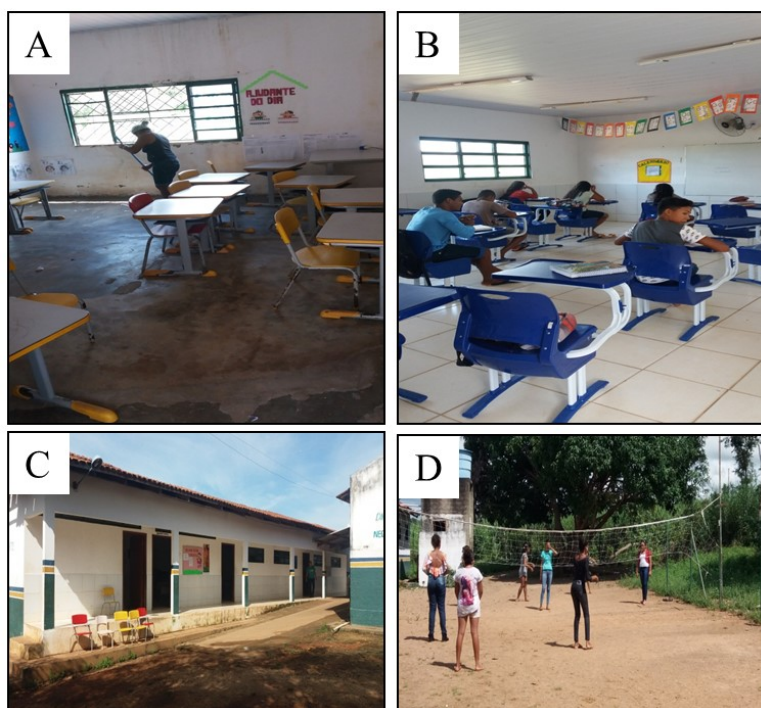
(A) Damaged classroom; (B) Preserved classroom; (C) Side view of the school; (D) Improvised space to play volleyball.
